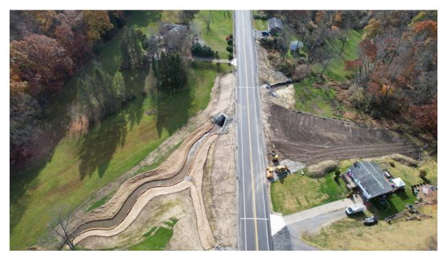
Photo 2: Newly constructed precast concrete box culvert carrying SR 356 over Tributary 2 to Kiskiminetas River
