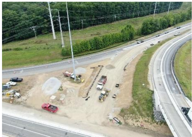
New Southbound I-95 ramp to Westbound 273 - During construction.
