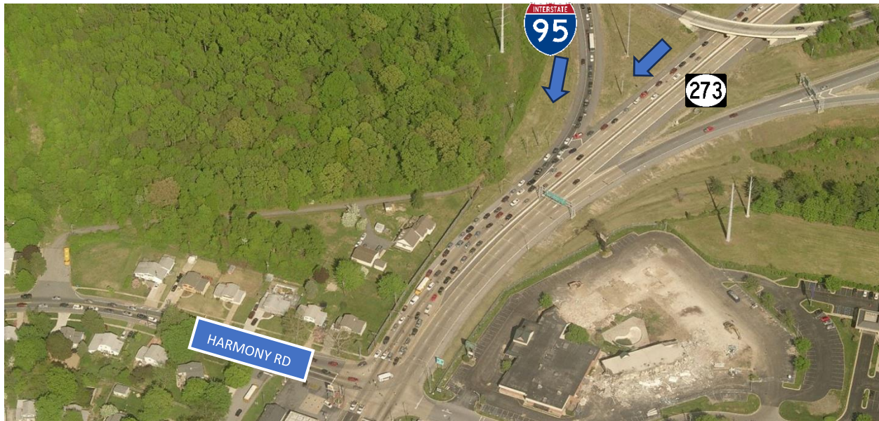
Pre-construction weaving condition.
