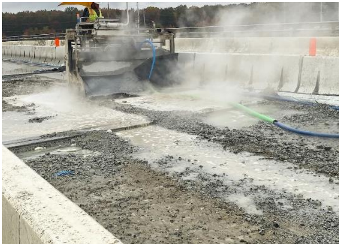
Bridge deck removal.
