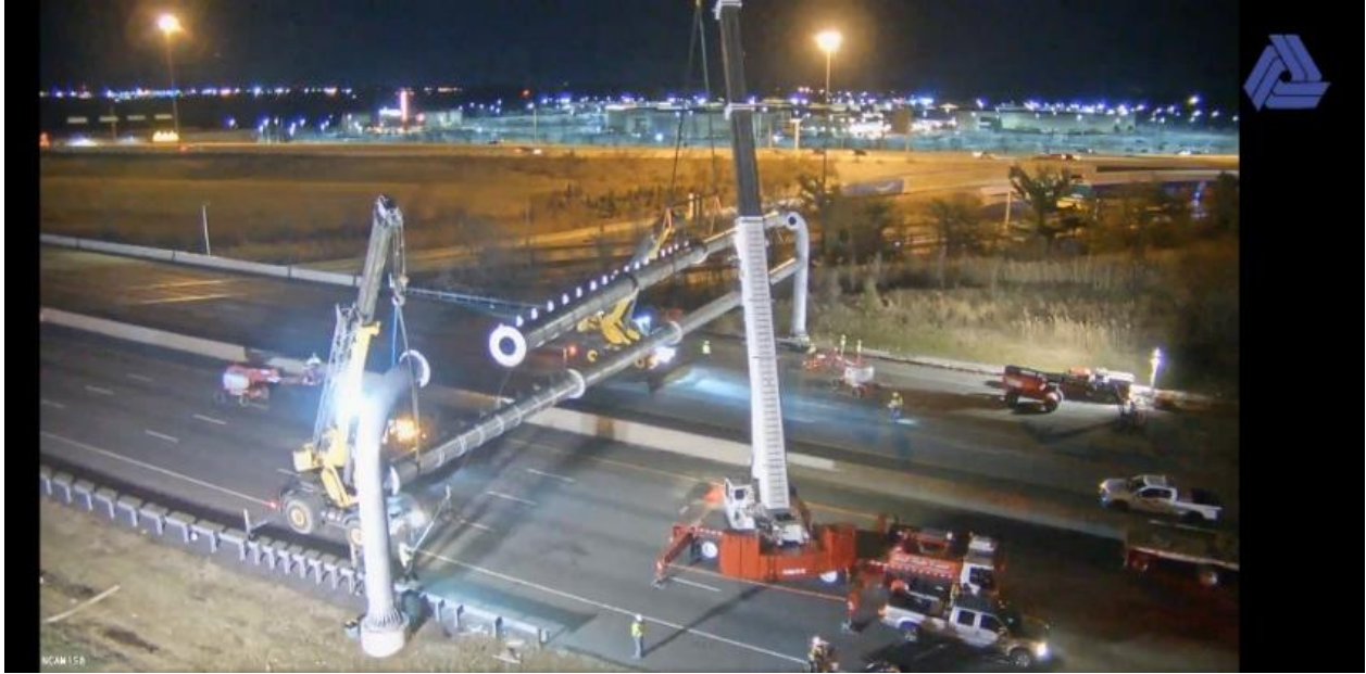
I-95 closure for overhead sign erection.
