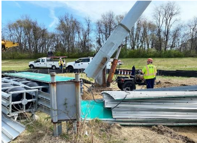
High mast lighting replacement.
