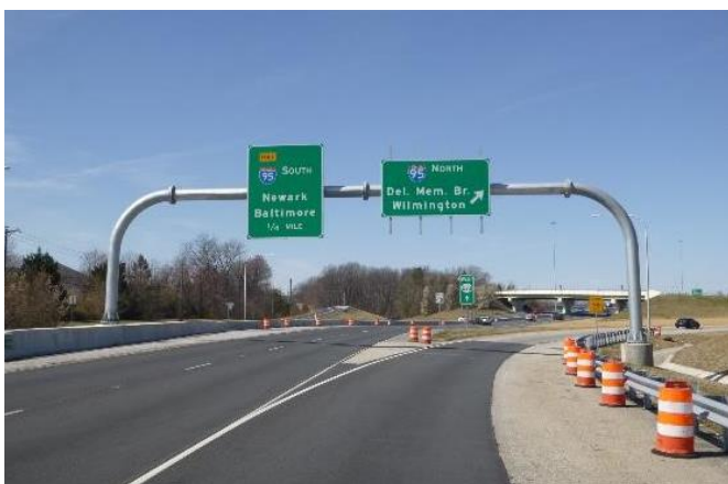
WB 273 overhead sign replacement.
