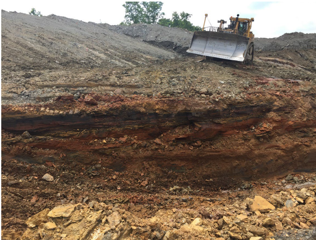
Photo 5 – 55A-1 Pickle Sludge Excavation
