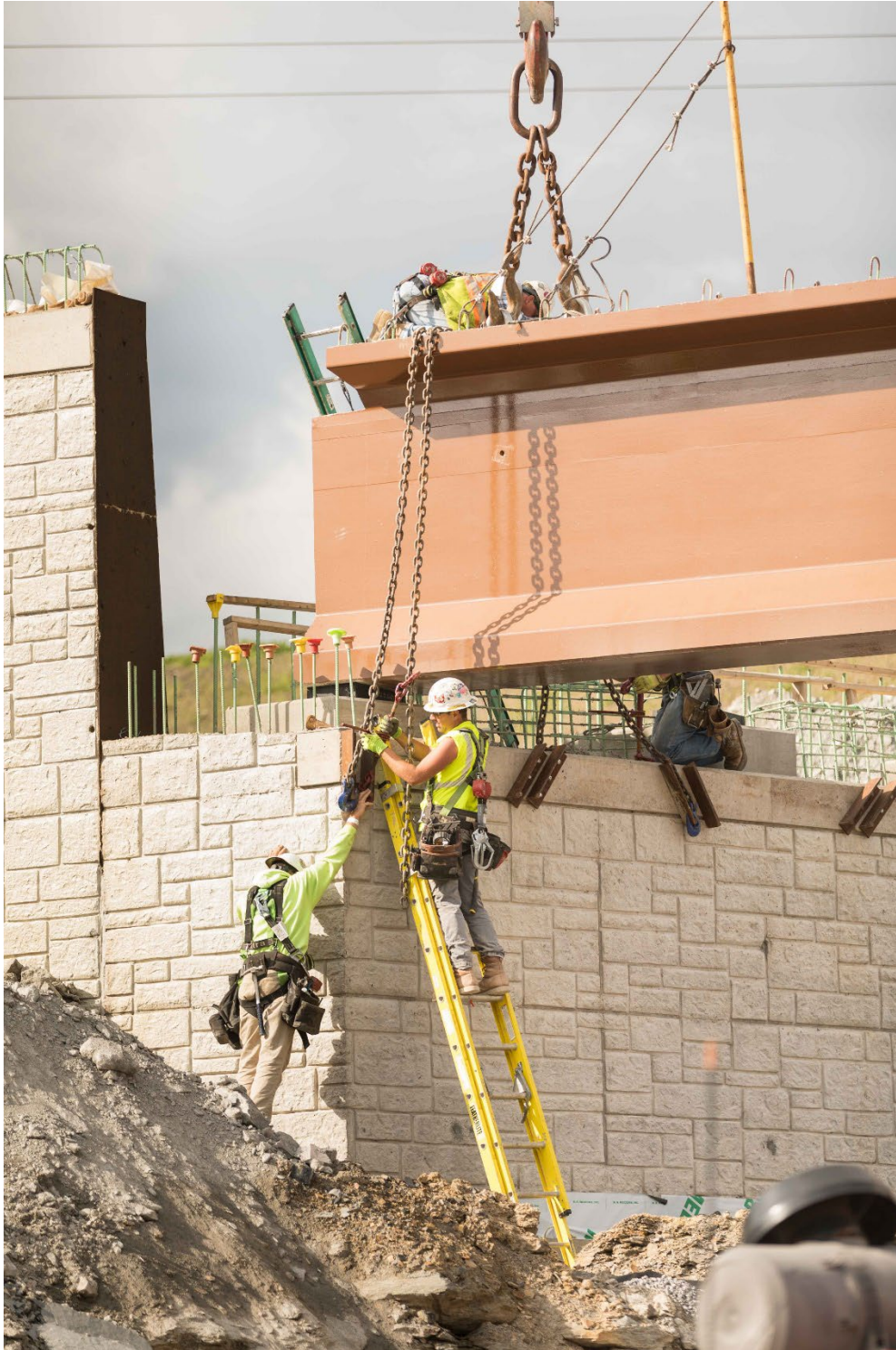
Photo 3 – Setting Bridge Beams
