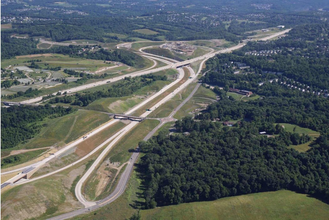
Photo 1 – Aerial View of Completed Interchange with Morganza Road
