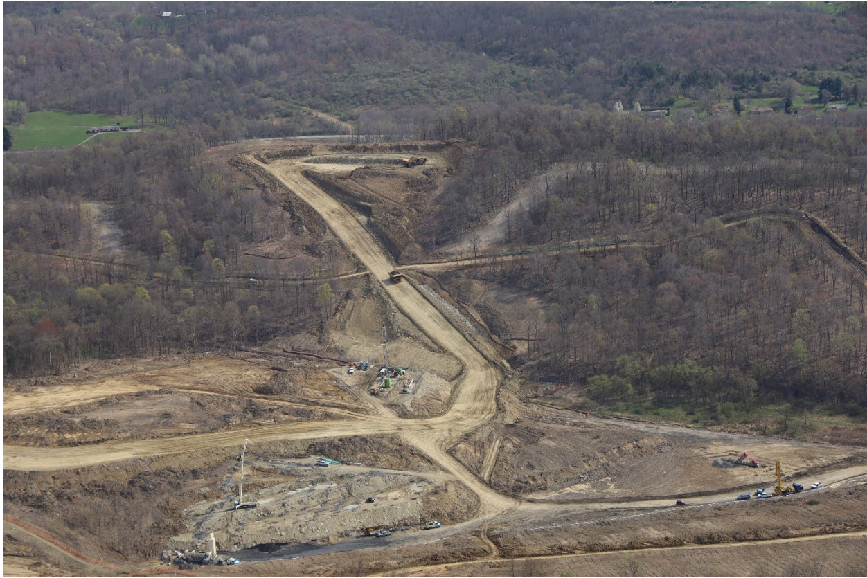
Photo 4 – Gas Well Plugging
